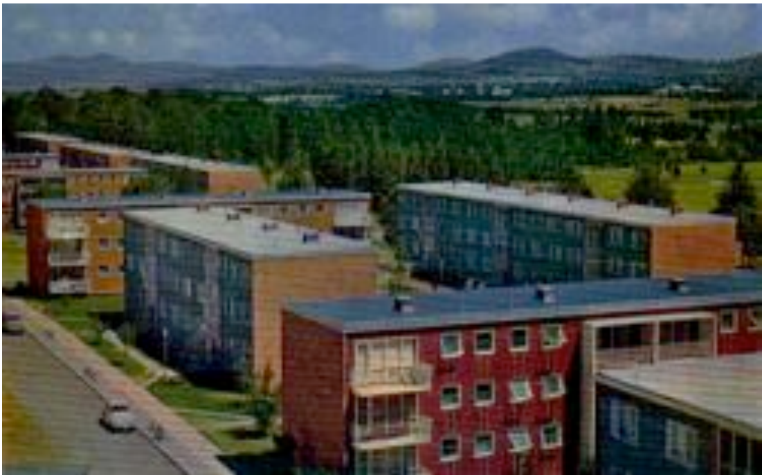
Illustration 1: Allawah and Bega Courts, c 1957, prior to construction of Currong Flats. From postcard reproduced at www.canberrahouse.com . 1
