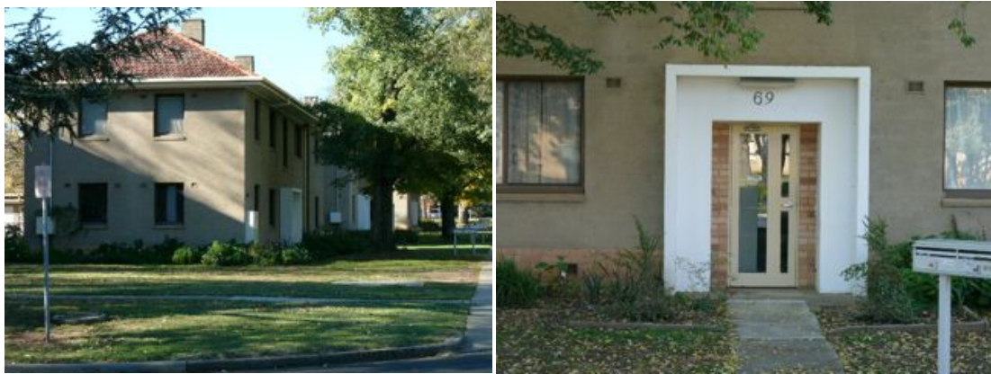
Illustrations 6 & 7: Braddon and Reid Flats. Photos by Milton Cameron, 2010.
