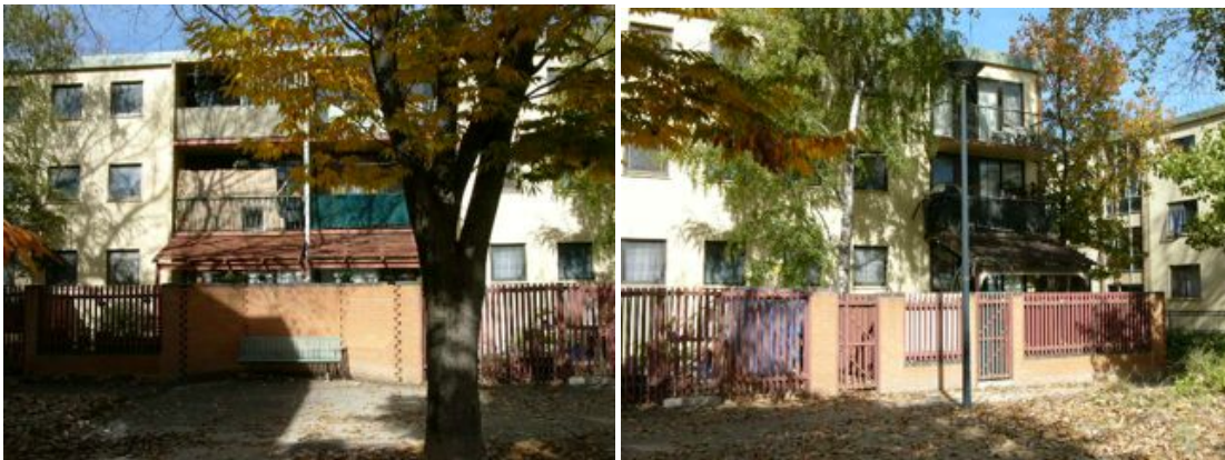
Illustrations 36 & 37: Allawah Courts showing later additions of walls, fences, gates, pergolas and improvised sun-screening and safety devices. Photos by Milton Cameron, 2010.
