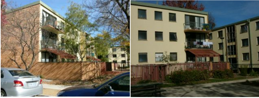
Illustrations 38 & 39: Allawah Courts showing later additions of walls, fences, gates, pergolas and improvised sun-screening and safety devices. Photos by Milton Cameron, 2010.
