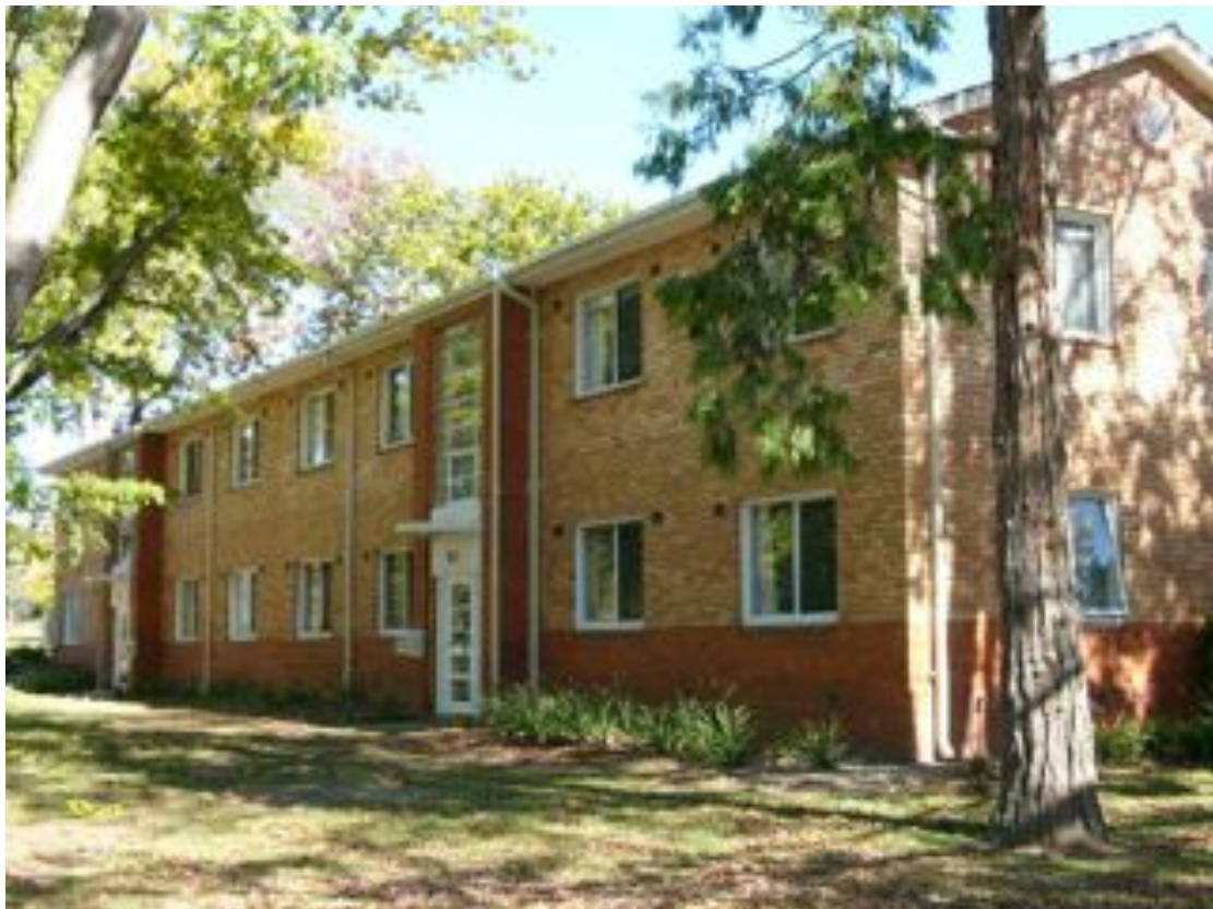
Illustration 3: Griffith Flats. Photo by Milton Cameron, 2010 .
